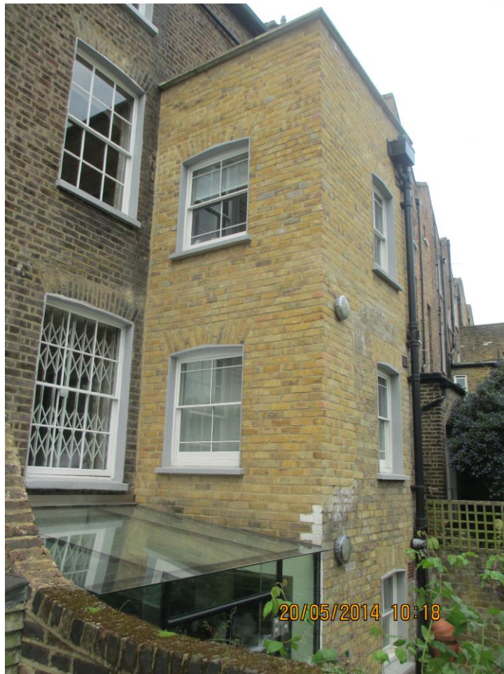
Image 3 – View of rear elevation of the adjoining property at no. 10 St Paul's Road
